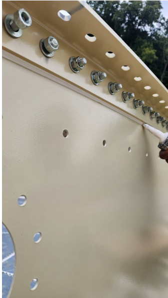
Photo 3 — Sealant being gunned along a horizontal lap during erection. The continuous bead is laid before the next sheet is set, then tooled into a fillet at the exposed edge.
