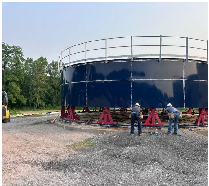
Photo 2 — Glass-fused-to-steel tank being jacked: the completed upper courses are raised and the next course is bolted in beneath them — the reverse of welded-tank erection.
