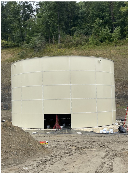
Photo 1 — Factory-coated (FBE) bolted shell during erection, before the roof and appurtenances are set. Note the staggered vertical seams and the temporary door sheet left out at the base for access.
