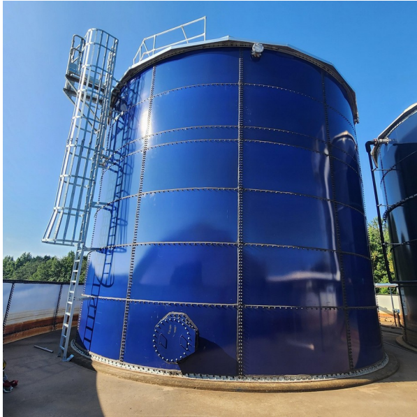
Photo 7 — Glass-fused-to-steel tank with exterior caged ladder, roof handrail and shell manway. The high-gloss cobalt finish is the fired glass itself; note the sealant fillets visible at every lap.
