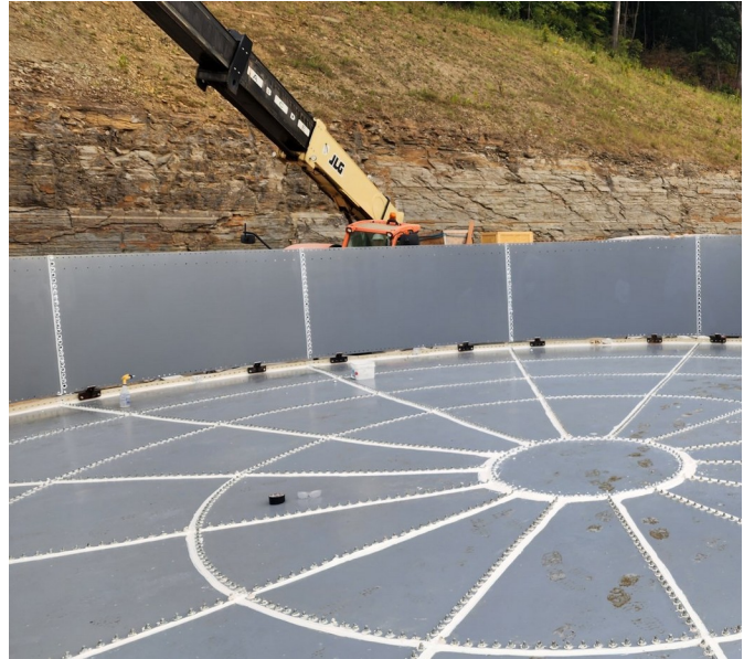
Photo 4 — Bolted steel floor with every radial and circumferential lap sealed and every bolt capped before the shell is raised; the base angle and hold-down clips are visible at the perimeter.
